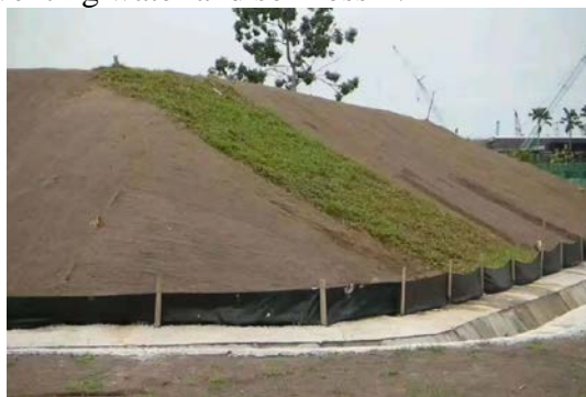
Fig.1 Ecological Vegetation Blanket Used for Slope Protection
